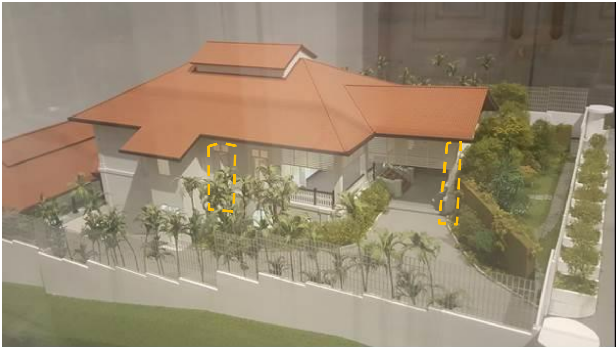
Left: Full length louvre windows (French windows) and Right: Classical column on plinth. Source: NHB.
