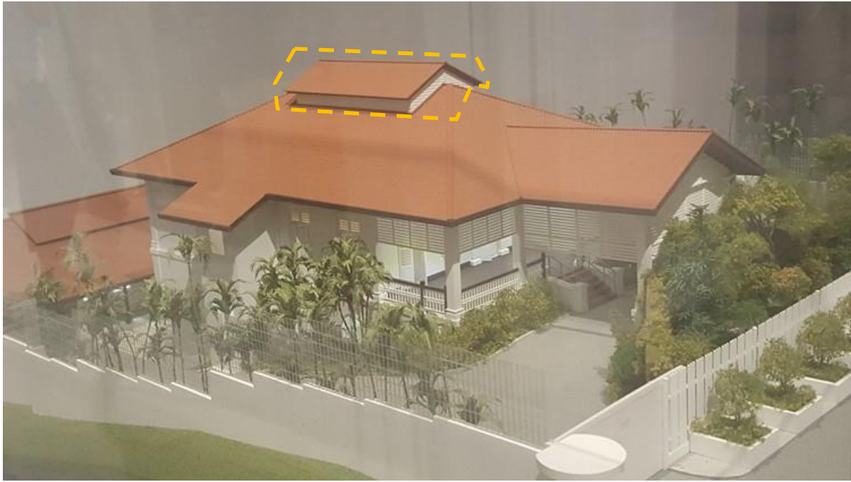
Jack roof of No. 38 Oxley Road. Source: NHB.
