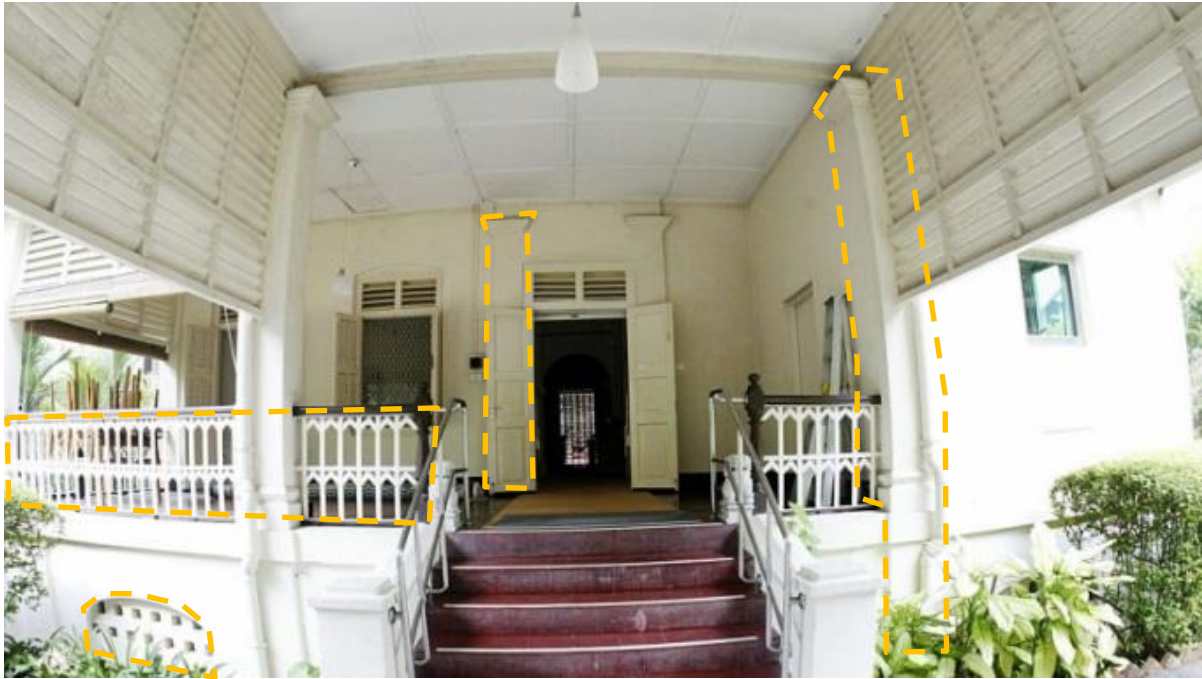
Bottom Left: Grilled vent for arched masonry; Left middle: Fretted Timber balustrades; and Middle and Right: Classical pilaster, columns and plinths
