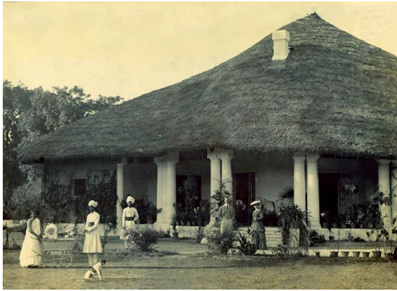
Anglo Indian Bungalow sitting on a low raised plinth. Source: Thatching Around the World... Around 1900. Accessed August 1, 2017. http://thatchinginfo.com/thatching-around-the-world-in-around-1900/ .
