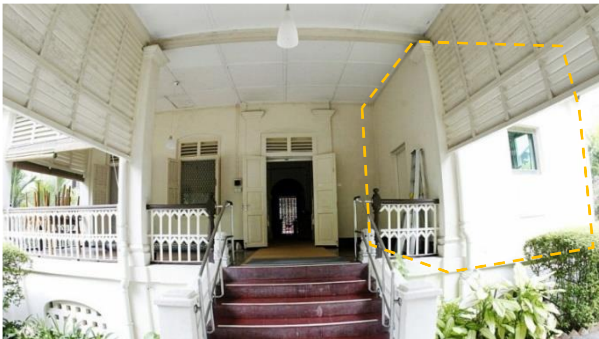
The verandah with part of it enclosed and converted into a room.
