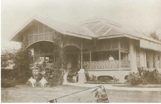
Photo of a Bungalow (circa 1900) – Reduced verandah, shorter overhanging eaves & wooden columns
